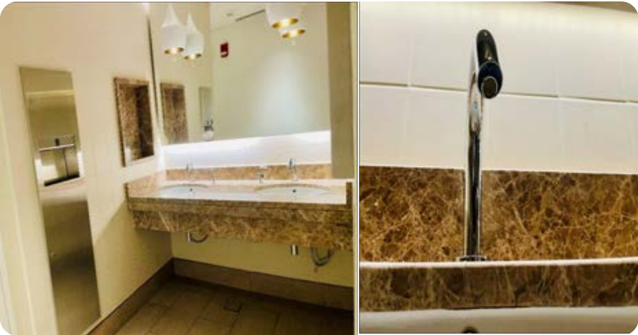
Faucet aerators have been installed in key facilities to minimize unnecessary water usage
